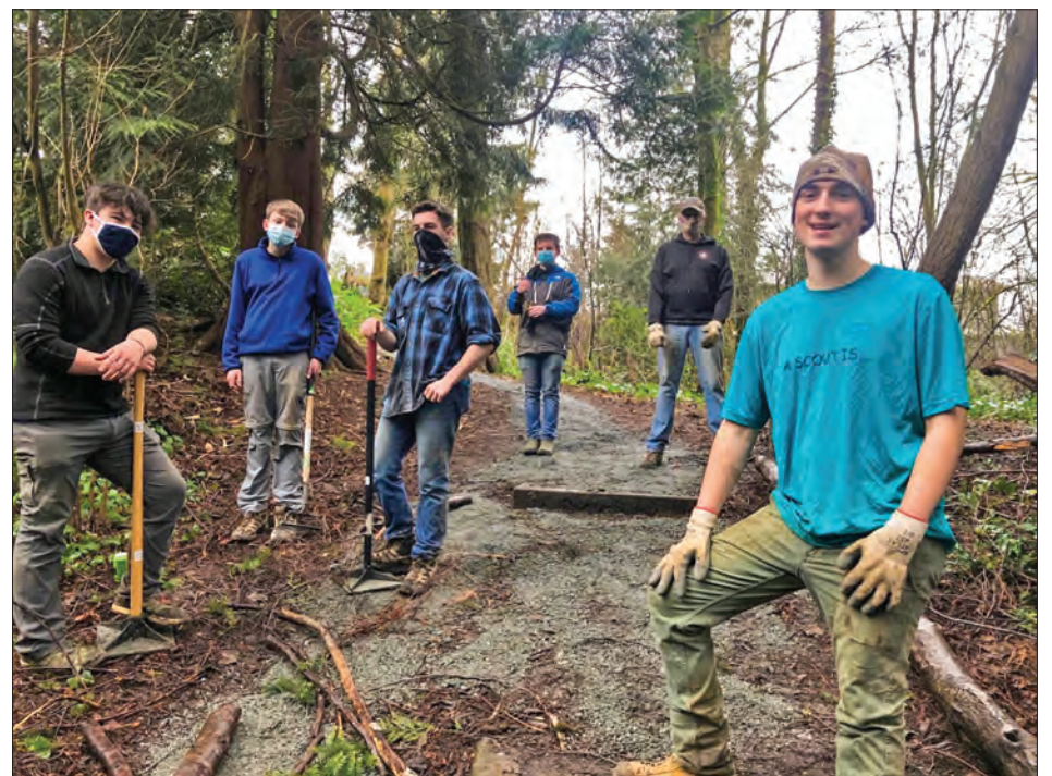
Noah Reid (right) and fellow scouts construct staircase at Pioneer Park.
