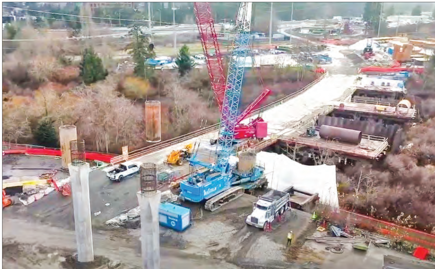
Construction progress on the L300 Lynnwood Link Extension project. Source: SkanskaUSA.
