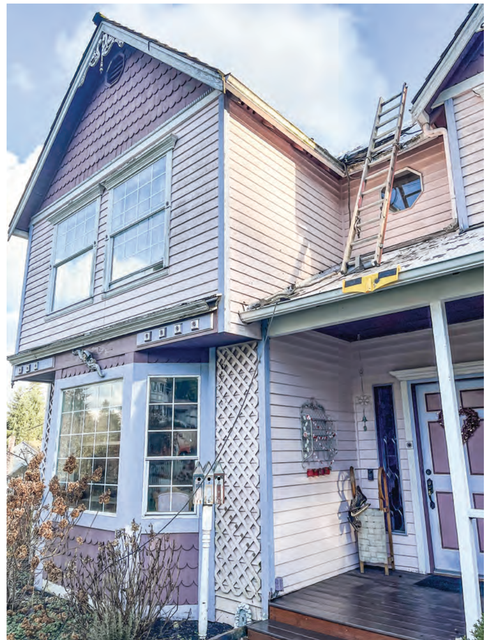
Brier Rose under repair by Habitat for Humanity. LT/Kienan Briscoe.
