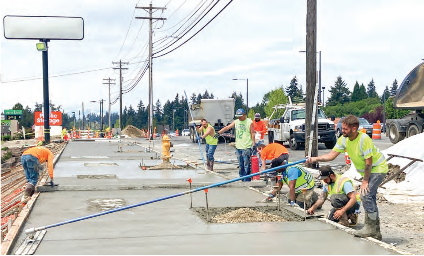
196th Street widening project taken on June 2, 2022. Source: Lynnwood Public Works.
