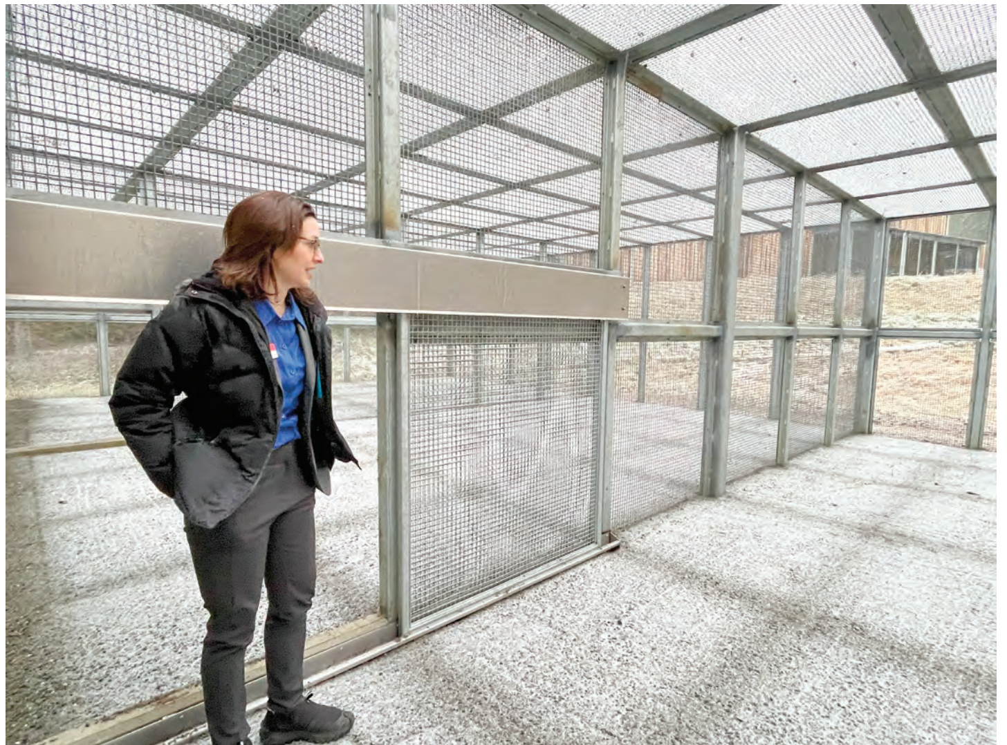
Heidi Willis, PAWS CEO, at the construction site of its upcoming wildlife center in Snohomish. SOURCE: Lynnwood Times | Kienan Briscoe.
